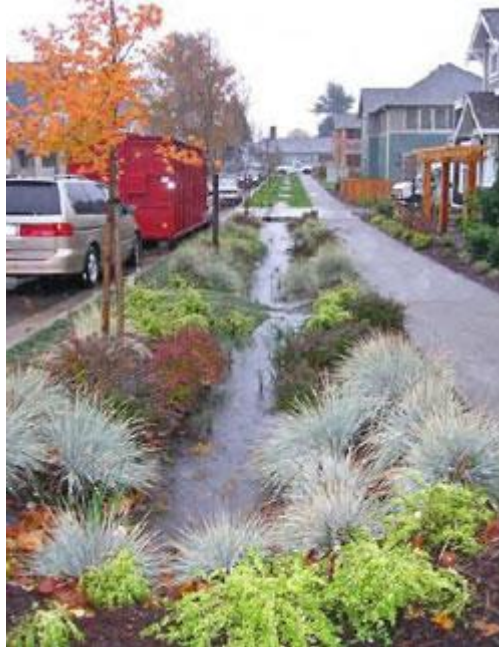
Water-filled planted swale during 25-year storm event
