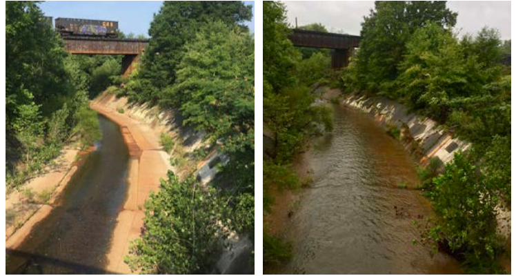
During periods of sparse precipitation, the Gillies Creek channel has a slow, low flow (left). During rain events, the water level rises quickly and water rushes through the concrete channel into the James River (right).
