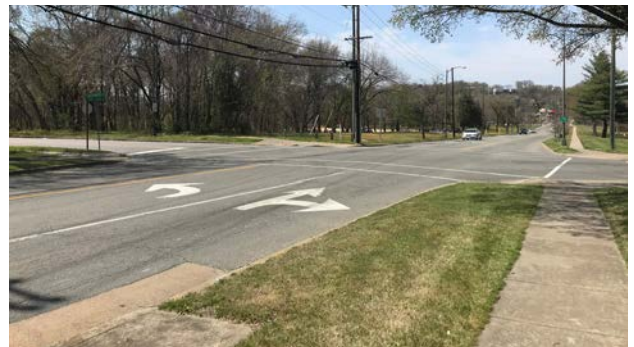
Runoff from Government Road can be diverted from street drains into planted curb extensions or swales.
