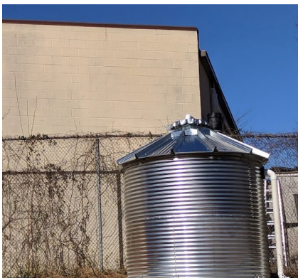
Water harvesting system installed to support large community garden.
