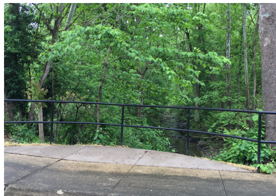
New creek overlook installed.
