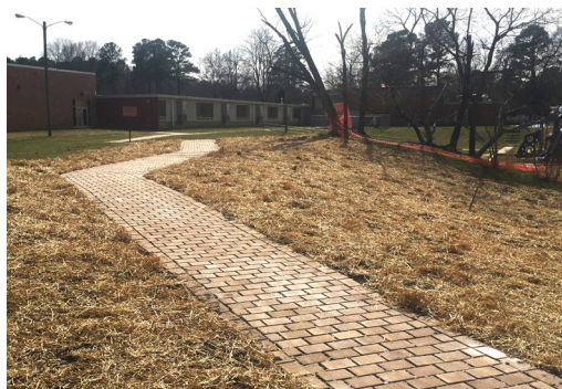
New trail connecting neighborhood to school using permeable pavers.
