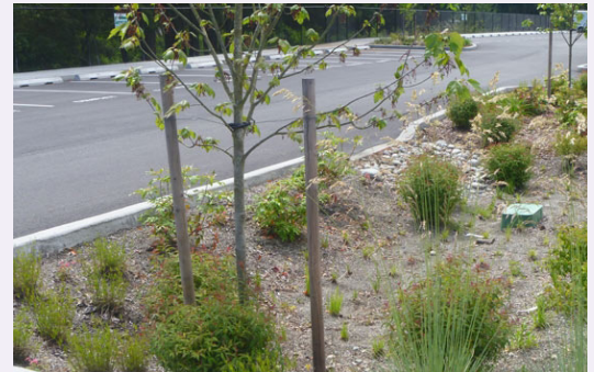
Parking lot infiltration island. Photo courtesy of The Watershed Company.
