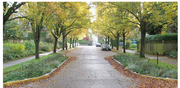
Example of stormwater bump-outs and road narrowing to slow traffic and treat stormwater runoff. Image source: ASLA.
