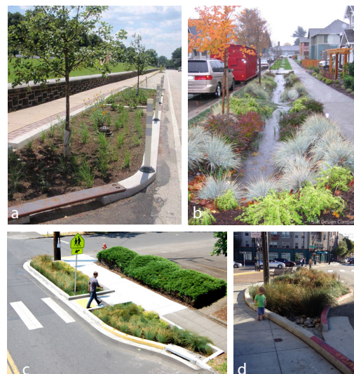
Examples of natural drainage strategies that support stormwater and walkability: a) curb extension, b) planted swale, c) curb extension with crosswalk, d) corner stormwater bulb-out with sidewalk.
