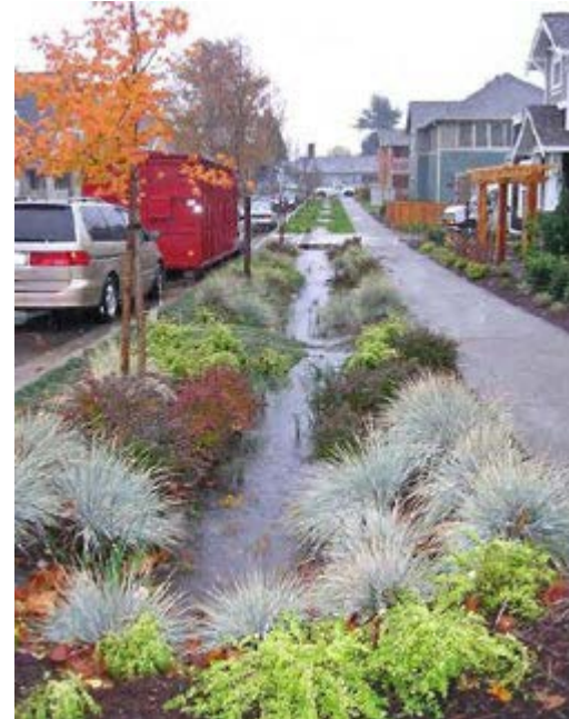
Water-filled planted swale during 25-year storm event
