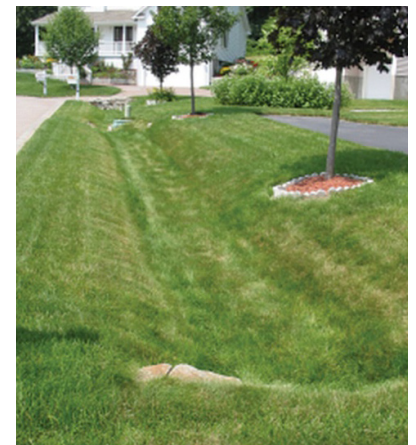
Example of how grassy swales along streets without sidewalks could address on-street flooding by providing holding space for stormwater during rain events.
