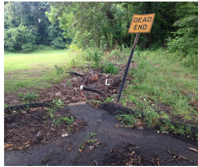
End of Light Street before rip-rap channel installed.
