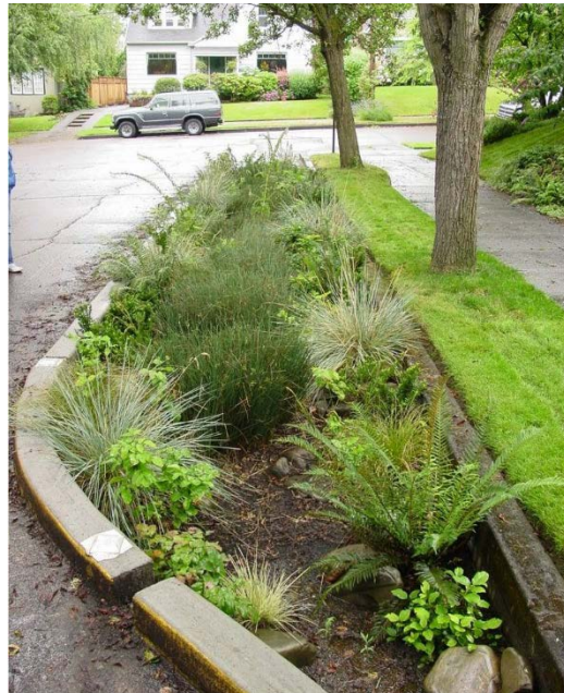
Curb extension retrofit
