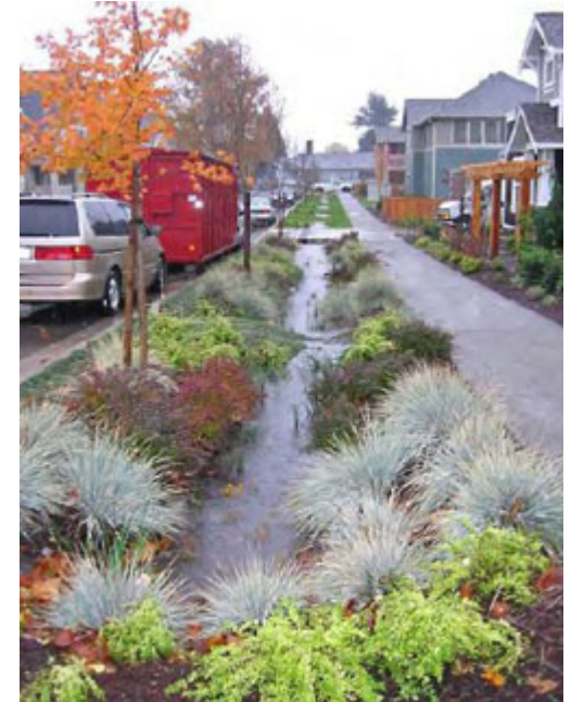
Water-filled planted swale during 25-year storm event
