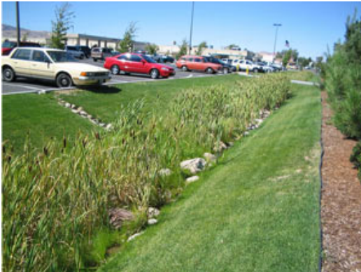
Vegetated swale at Costco parking lot Photo courtesy of Sue Donaldson.
