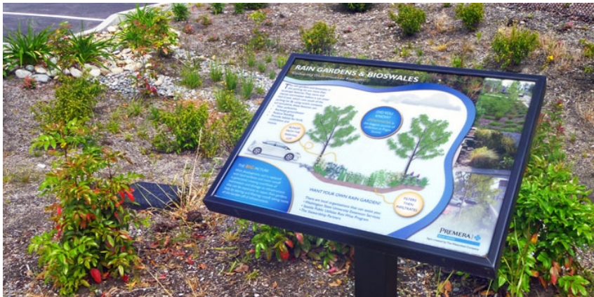
Parking lot infiltration island with signage. Photo courtesy of The Watershed Company.
