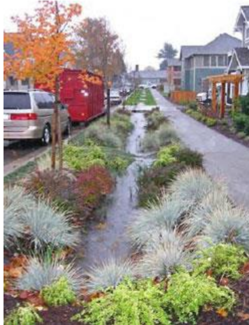
Water-filled planted swale during 25-year storm event
