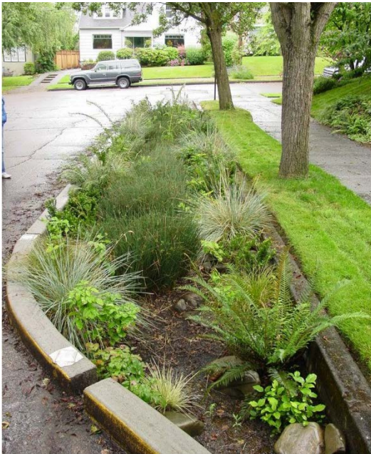
Curb extension retrofit
