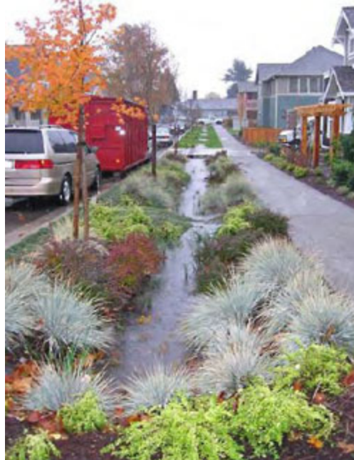
Water-filled planted swale during 25-year storm event
